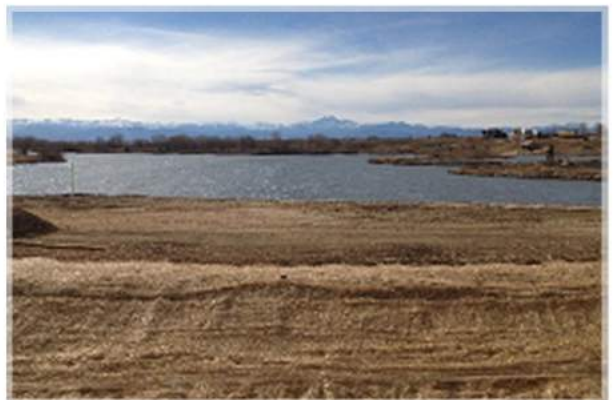
March 2014- area repaired, and blanket set to protect from erosion
