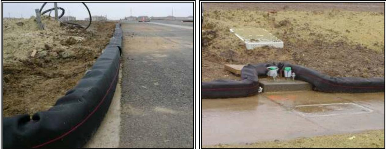
**The Heavyweight™ Wattle** provides a practical alternative to a straw wattle or silt fence that will rebound to its original shape time and time again. Simply put, you can run it over with just about anything up to hundreds of times and it keeps its shape. The wattle is almost impossible to undermine and the barrier maintains an effective height under the worst of conditions and elements.
